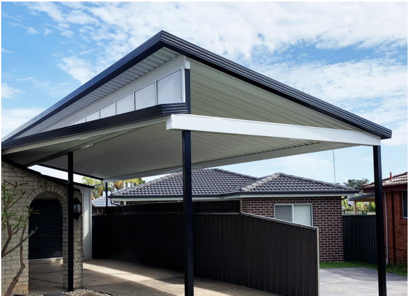
Flyover Carport featuring the Allform Roof Profile, Beams and Gutter.
